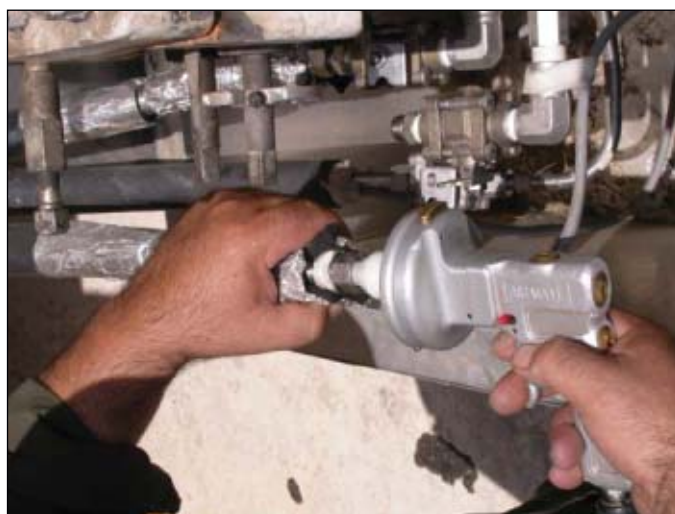
A pellet launcher (left) removed black powder from gas metering impulse lines. The pellets used (right) turned black after just one pass through the impulse line (Fig. 7).
